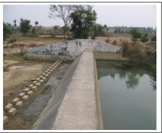
To facilitate smooth flow of approaching floodwaters towards the weir, the upstream area of the weir is cleared for the required width and to the levels, to prevent heading up of water that may cause overtopping of the embankment.
