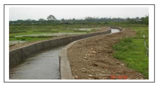
The conveyance channels have minor masonry structures such as outlets structures with or without controlling gates, cattle crossings, cart track crossings, cross drainage works crossing valleys, canal drops etc. to safely carry the channel flow to the tail end of the command area.
