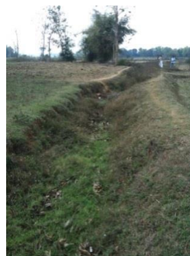
(d) Unlined canal section at tail of the same system. No uniform shape, high seepage losses and unable to maintain command at outlets, OCTMP, Odisha.
