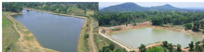
Figure-6.6:Water Harvesting Tanks/WDS
